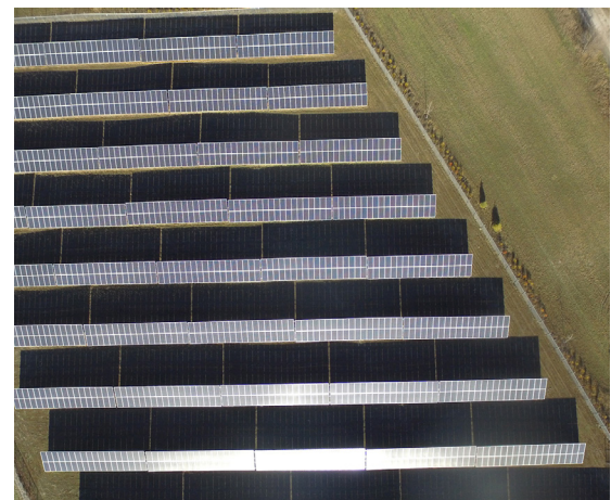
Project MC-ML81, a 600kW DC ground mount solar project.
